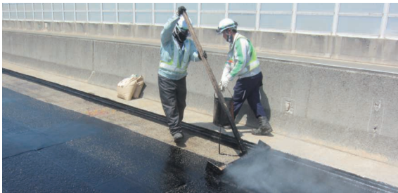
Construction in progress
