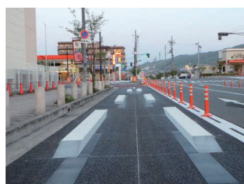
Road markings that appear to be three-dimensional
