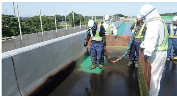
Construction in progress
