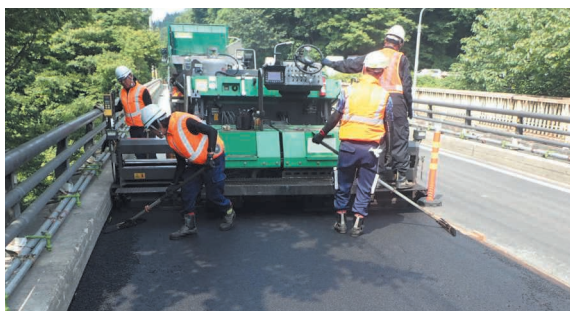
Construction in progress
