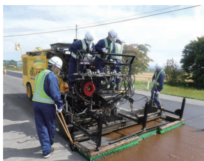
Leveling with a specialized vehicle
