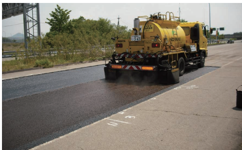
SUPER TACKZOL with immediately breaking even at night or at low temperatures and firm adhesion of pavements
