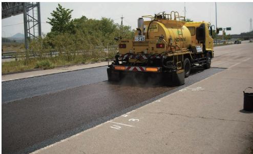
SUPER TACKZOL with immediately breaking even at night or at low temperatures and firm adhesion of pavements
