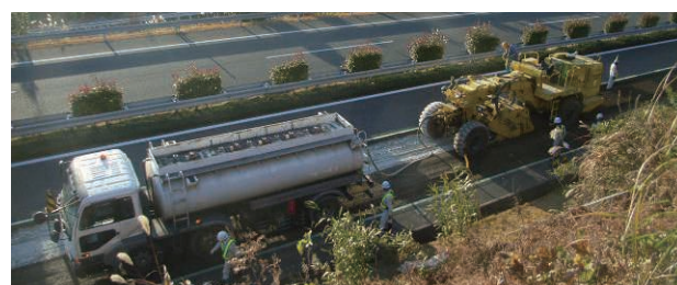
STABI-CEMENT RC construction method (mixing method with a deep stabilizer) Cement and asphalt emulsion stabilizing base course construction method (on-site base course recycling construction method) in which the road's existing asphalt mixture and the base course are crushed and mixed at the same time with asphalt emulsion and cement
