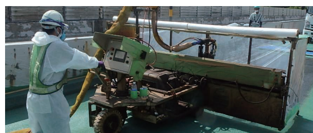
HQ HIBRANE AU construction method (construction with a binder spraying robot) Highly durable asphalt urethane membrane type waterproofing method for bridge deck slab, assuming a design durability of 30 years
