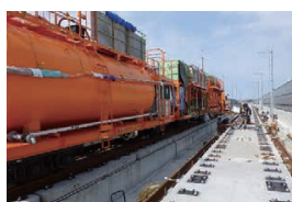
CA mortar filling construction method (Shinkansen slab track filling construction method)
