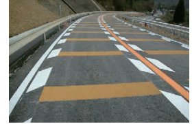
COALCUT R construction method (resin-based anti-skid paving)
