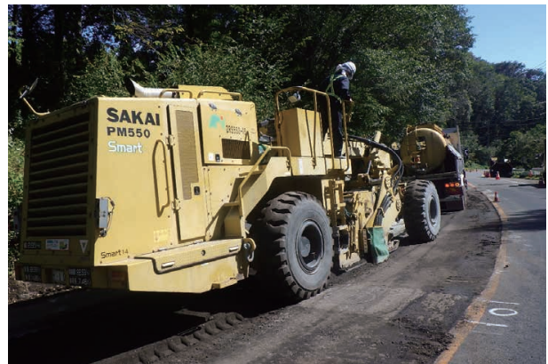
STABI-CEMENT RC construction method (mixing with a road stabilizer)
