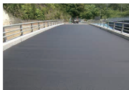
SUPER SURFTREAT construction method (asphalt emulsion surface treatment construction method)
