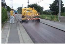
SUPER TACKZOL (rapid breaking asphalt emulsion)
