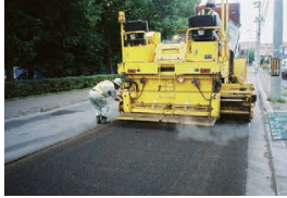
EMULTEC SAMI construction method (crack prevention cushion layer construction method)
