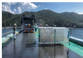
HQ HIBRANE AU construction method (high-performance bridge deck slab waterproofing method)
