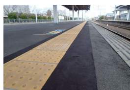
SUPER ROMENPATCH (cold curing bump repairing material)
