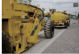
STABI-CEMENT RC construction method (on-site base course recycling construction method)
