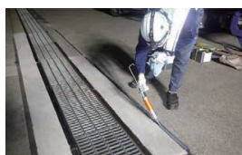
NEOTAIYU SEALCOLD (oil-resistant joint sealant)
