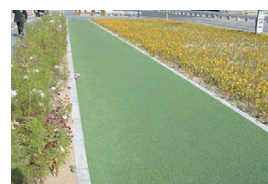
COALCUT R construction method (resin-based anti-skid paving)
