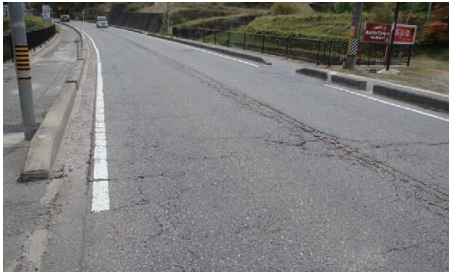
Damaged road pavement
