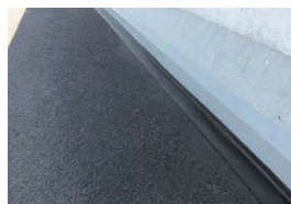
L-seal tape (molded water cut-off material for bridge ends)
