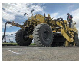
6 STABI-CEMENT RC construction method with road stabilizers using ICT technology
