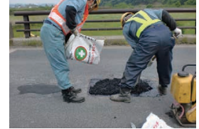
RESCUEPATCH (high durability, all-weather type cold applied patching material)
