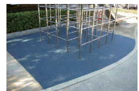
COLORPHALT DA construction method (rubber chip paving)
