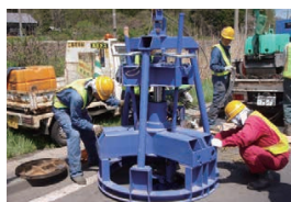
MR² method (manhole top repairing method)
