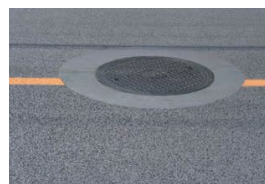
SUPER ROMENPATCH (cold curing bump repairing material)
