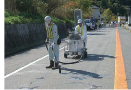
CRACKSEAL NX (hot applied crack sealant)
