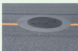
SUPER ROMENPATCH (emulsion based cold mix bump repairing material)
