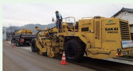
STABI-CEMENT RC construction method (on-site base course recycling construction method)
