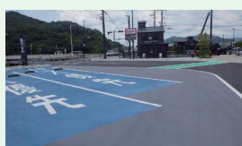
THERMOTEC construction method (heat-blocking paving)
