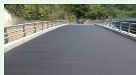
SUPER SURFTREAT construction method (asphalt emulsion surface treatment construction method)
