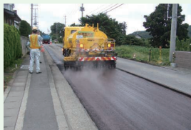
SUPER TACKZOL (rapid breaking asphalt emulsion)
