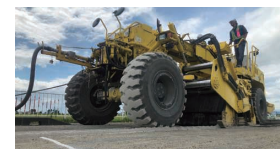
Construction with a road stabilizer
