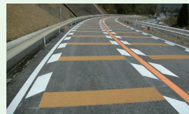
COALCUT R construction method (resin-based anti-skid paving)
