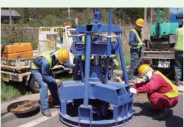
MR² method (manhole top repairing method)
