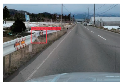
Damage to a guardrail
