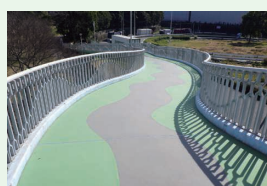
COLORPHALT KT method (resin mortar based color paving)
