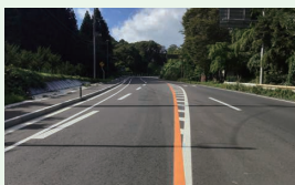
SHINAYAKAPHALT (modified asphalt for long-lasting paving)
