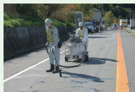
CRACKSEAL NX (hot applied crack sealant)
