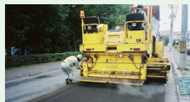
EMULTEC SAMI construction method (crack prevention cushion layer construction method)
