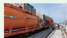
CA mortar filling construction method (Shinkansen slab track filling construction method)
