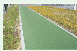
COALCUT R construction method (resin-based anti-skid paving)
