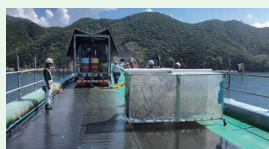
HQ HIBRANE AU construction method (high-performance bridge deck waterproofing method)
