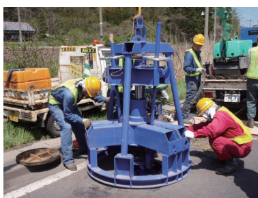
During construction (removal of a manhole)
