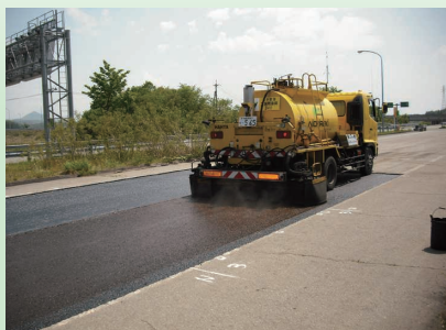
Rapid breaking asphalt emulsion SUPER TACKZOL
