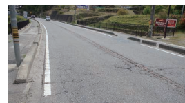
Damaged road pavement
