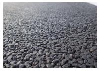
Pavement using small-particle size porous asphalt mixture (5)
