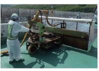
HQ HIBRANE AU construction method using a binder spraying robot
