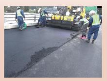
Pavement waterproofing method HQ PAVERANE construction method
