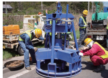
During construction (removal of a manhole)
