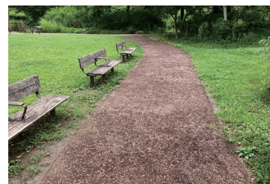
ASWOOD paving using trees damaged by Japanese oak wilt disease
