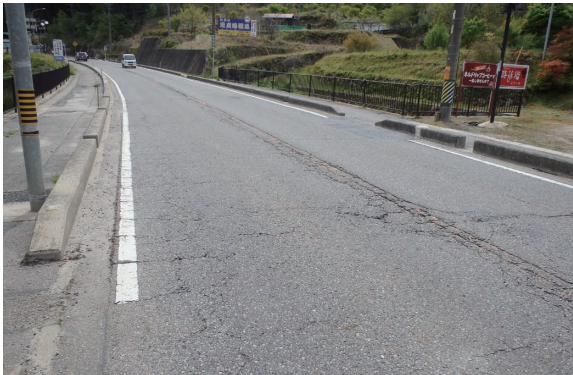
Damaged road pavement
