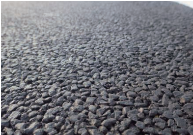
Pavement using small-particle size porous asphalt mixture (5)
