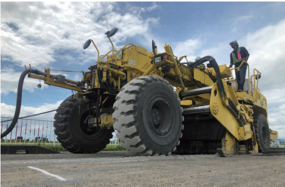
Construction with a road stabilizer
