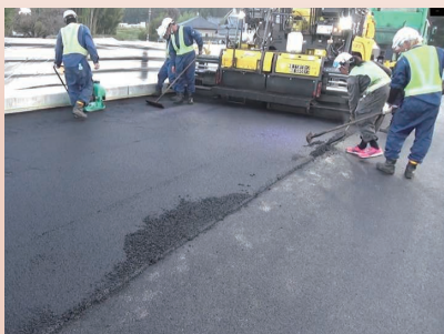
Pavement waterproofing method HQ PAVERANE construction method
