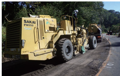
STABI-CEMENT RC construction method using ICT
