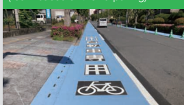
COALCUT R construction method (resin-based anti-skid paving)
