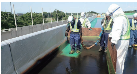
Construction in progress
