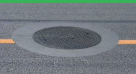
SUPER ROMENPATCH (emulsion-based cold mix bump repairing material)
