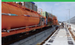
CA mortar filling construction method (Shinkansen slab track filling construction method)
