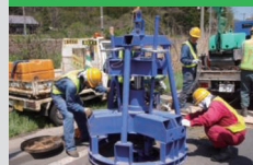
MR 2 method (manhole top repairing method)
