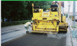
EMULTEC SAMI construction method (crack prevention cushion layer construction method)
