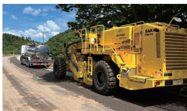
STABICEMENT RC construction method using ICT
