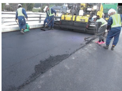
Pavement waterproofing method HQ PAVERANE construction method
