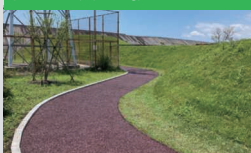
ASWOOD paving (wood chip paving)
