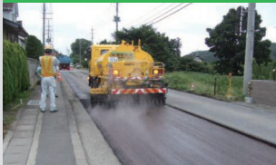
SUPER TACKZOL (rapid breaking asphalt emulsion)
