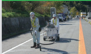
CRACKSEAL NX (hot applied crack sealant)
