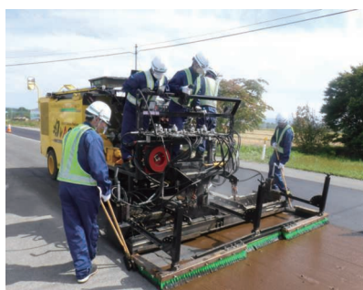
Leveling with a specialized vehicle
