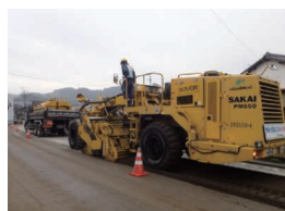
6 STABI-CEMENT RC construction method with road stabilizers using ICT
