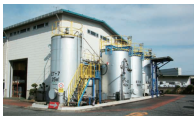
Chiba Manufacturing Plant
