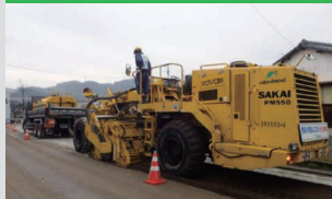
STABI-CEMENT RC construction method (on-site base course recycling construction method)
