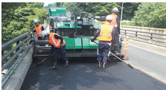
Construction in progress
