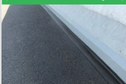
L-seal tape (molded water cut-off material for bridge ends)
