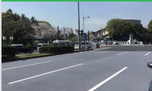
THERMOTEC construction method (heat-blocking paving)
