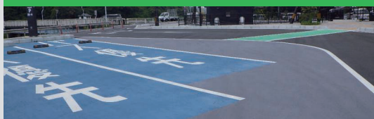
THERMOTEC construction method (heat-blocking paving)
