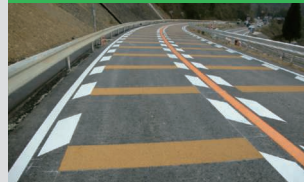
COALCUT R construction method (resin-based anti-skid paving)
