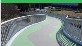
COLORPHALT KT method (resin mortar-based color paving)
