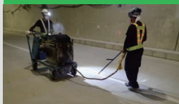
SEROSEAL (hot applied joint sealant for concrete joints)
