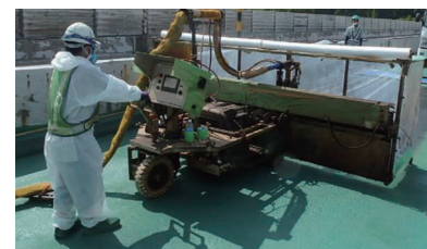
HQ HIBANE AU construction method using a binder spraying robot
