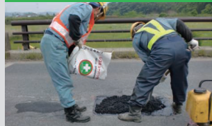
RESCUEPATCH (high durability, all-weather type cold applied patching material)
